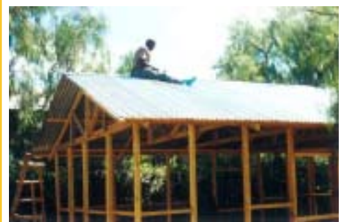
A temporary kitchen is under construction
